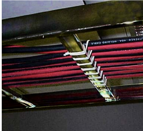
FIGURE 9-17 TELEPHONE COMPANY LACING METHODS
